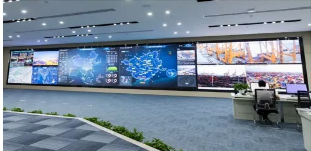
SOC Video Wall – Example (After)
